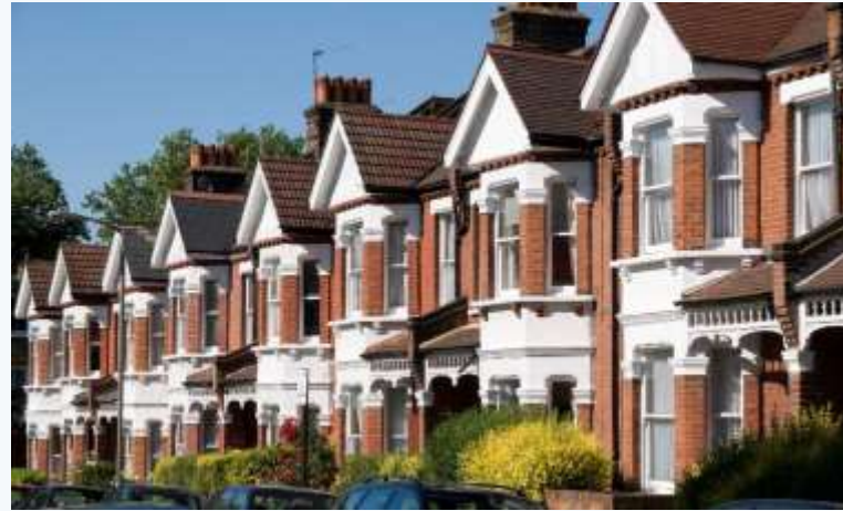
a terraced house
